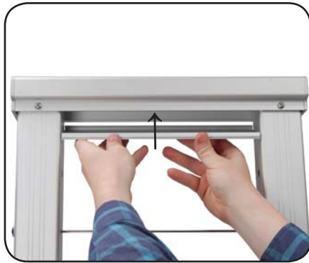
Series 200 - Flat Infill Cut flat infill to length and snap into bottom side of top rail. Install prior to tensioning the cables.
